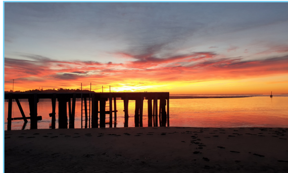
BARWON COAST AS THE MANAGER OF THE LOCAL PORT OF BARWON HEADS ON BEHALF OF THE DEPARTMENT OF TRANSPORT HAVE RECENTLY OVERSEEN MAINTENANCE WORKS ON THE MAIN PUBLIC JETTY DECK.
