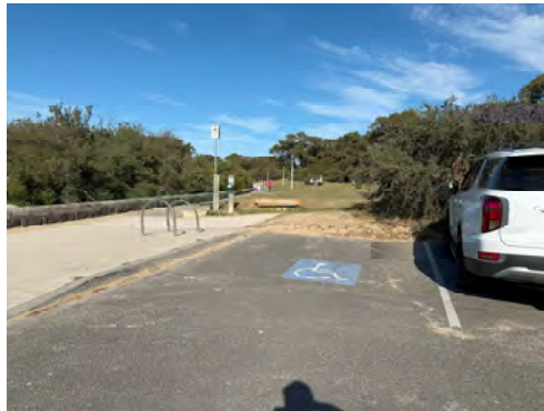
(c) No kerb ramp at accessible parking bay
