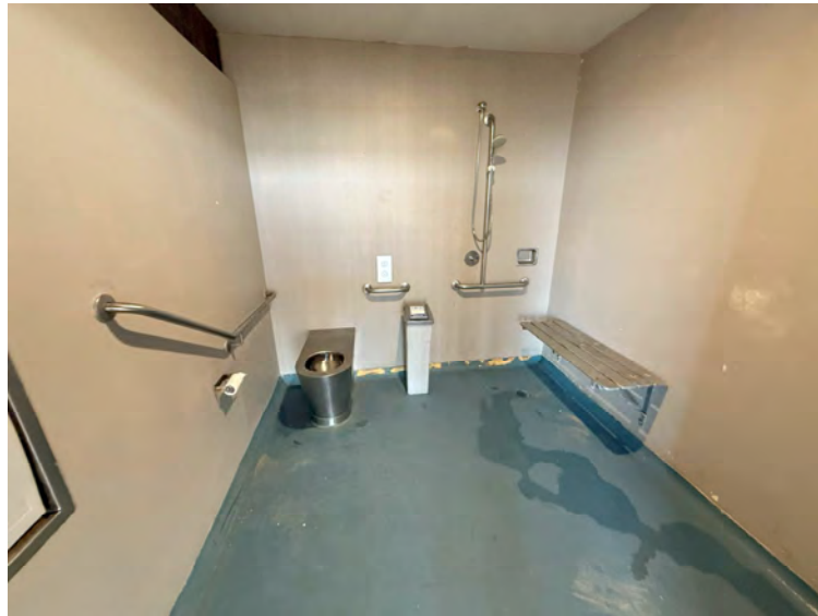
Figure 22: Current accessible bathroom Ocean Grove Main Beach
