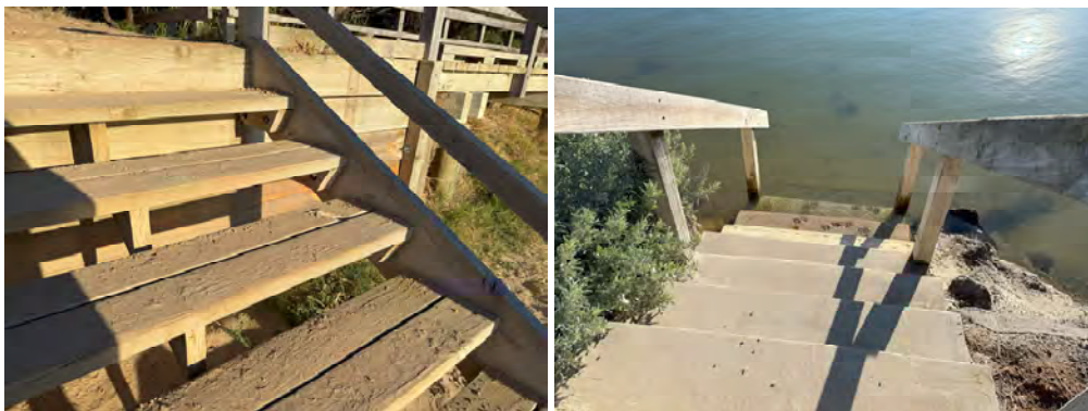
Figure 18: (a) Stairs at Ocean Grove boardwalk near bridge (b) Stairs to access river Ocean Grove side
